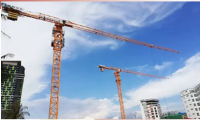
Hammerhead tower cranes
